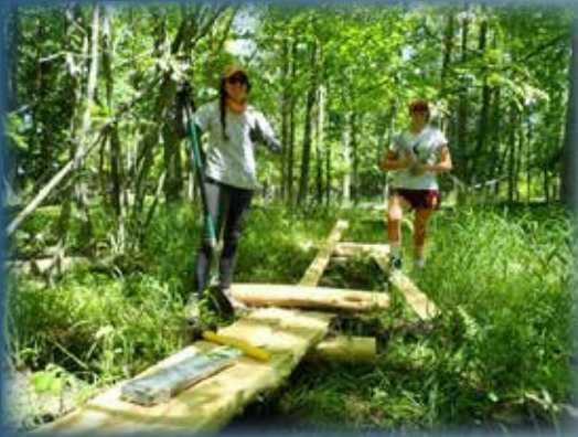
New puncheon installed at Hiawatha Hills Preserve
