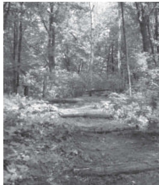
Erosion Control Measures
